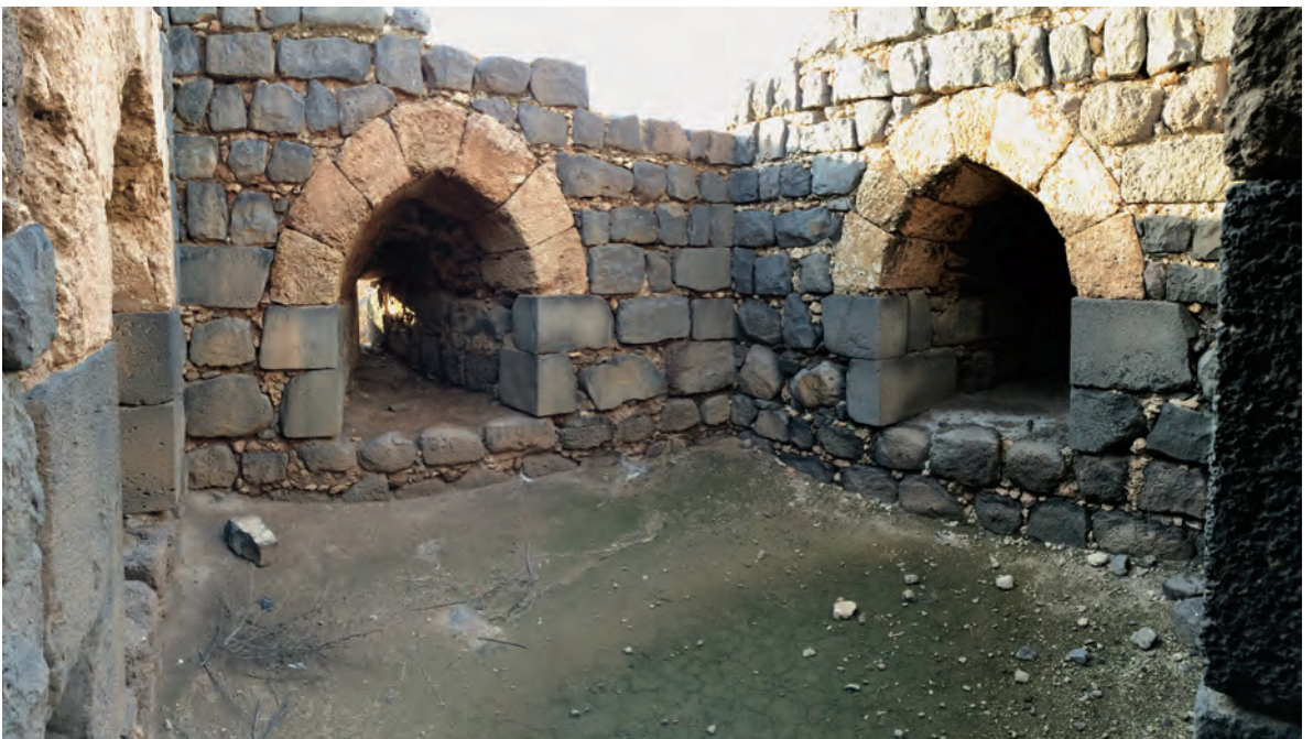
Belvoir, embrasures of one of the inner towers. (Michael Fulton)
